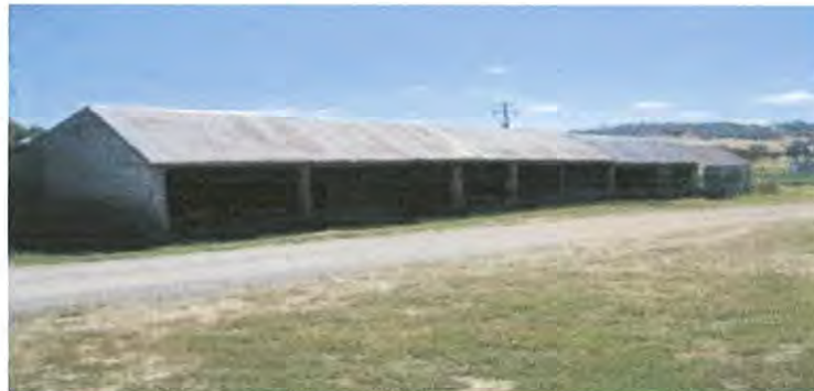
Figure 12 Facing north east showing the oldest of the study areas structures.
