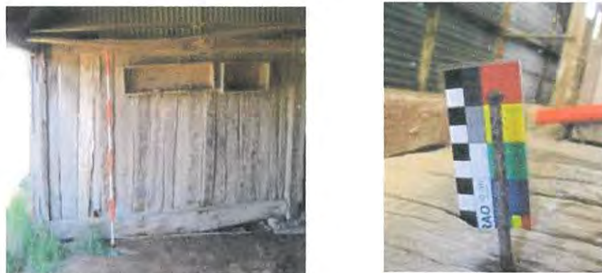
Figure 13 Showing split log wall (on left) and a 1890-1930 wire Romboïd nail (on right).
