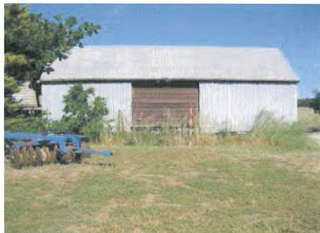
Figure 11 Facing west showing the general storage shed numbered as '2' within the study area.
