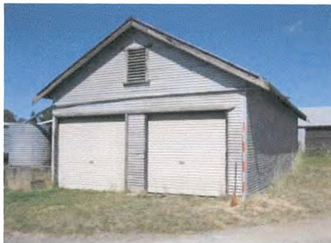
Figure 15 Facing south west to view the structure recorded as building 5 within the study area.
