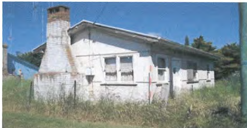
Figure 17 Facing south west showing the rectangle shaped construction numbered as Historical Site 7 within the study area.
