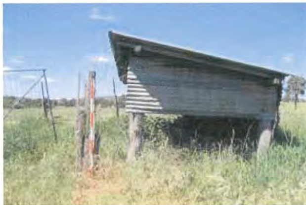
Figure 20 Facing south looking at the dilapidated chicken pen located within the study area.
